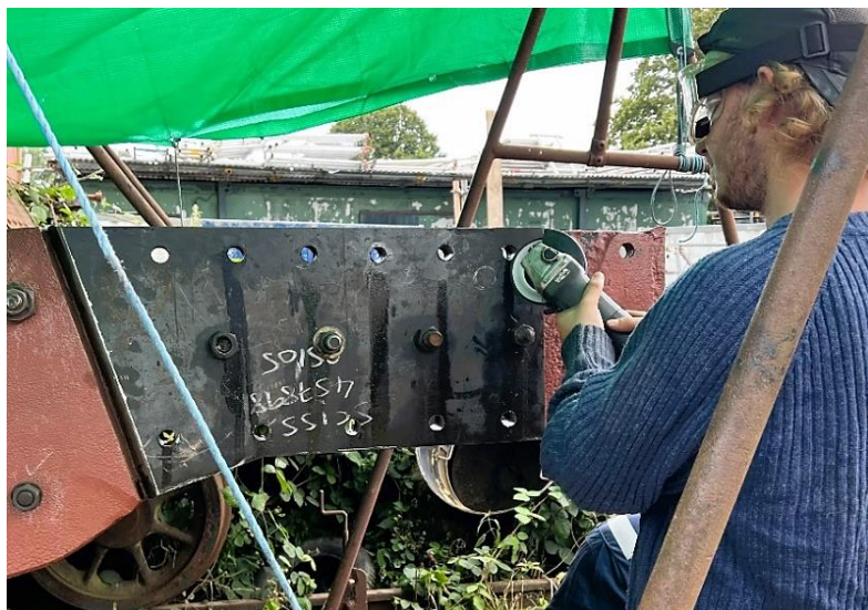
Harry Highman cleans up the new steel section prior to welding
